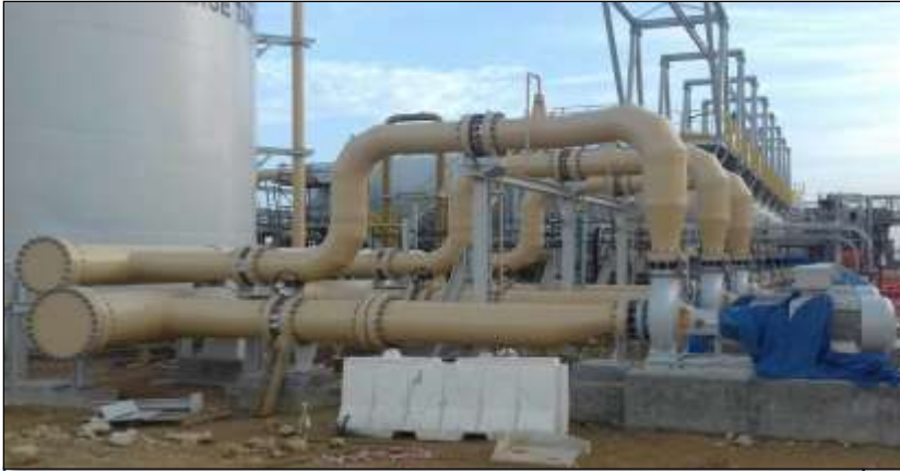
GRP Piping Fabrication & Erection Works in Backwash Area
