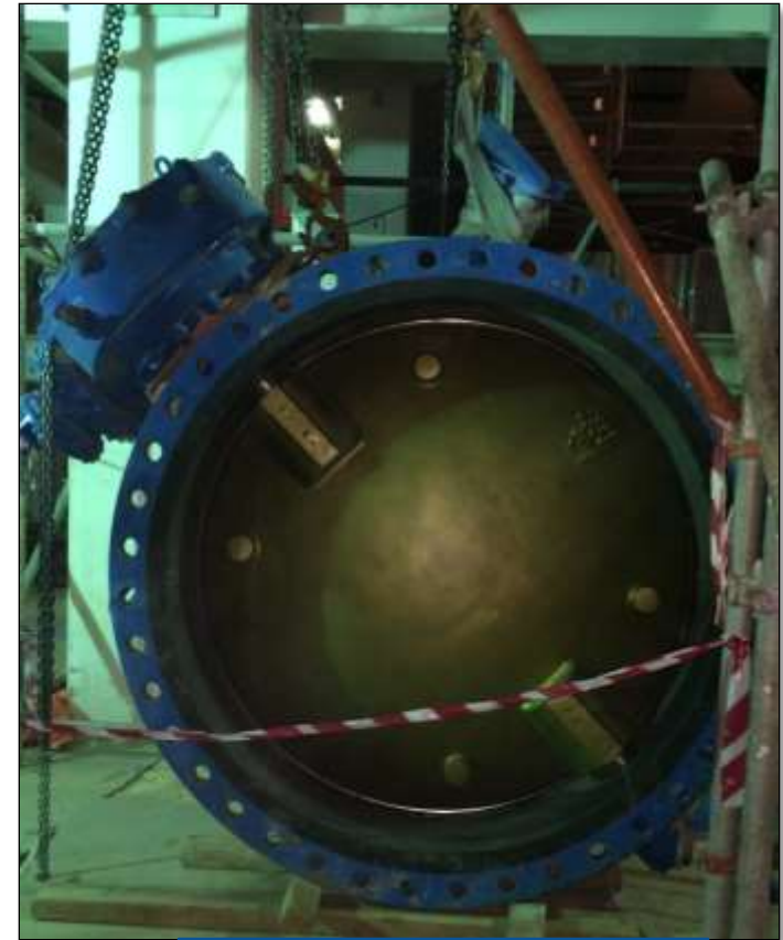
Erection of Valves at Energy Center Pump House
