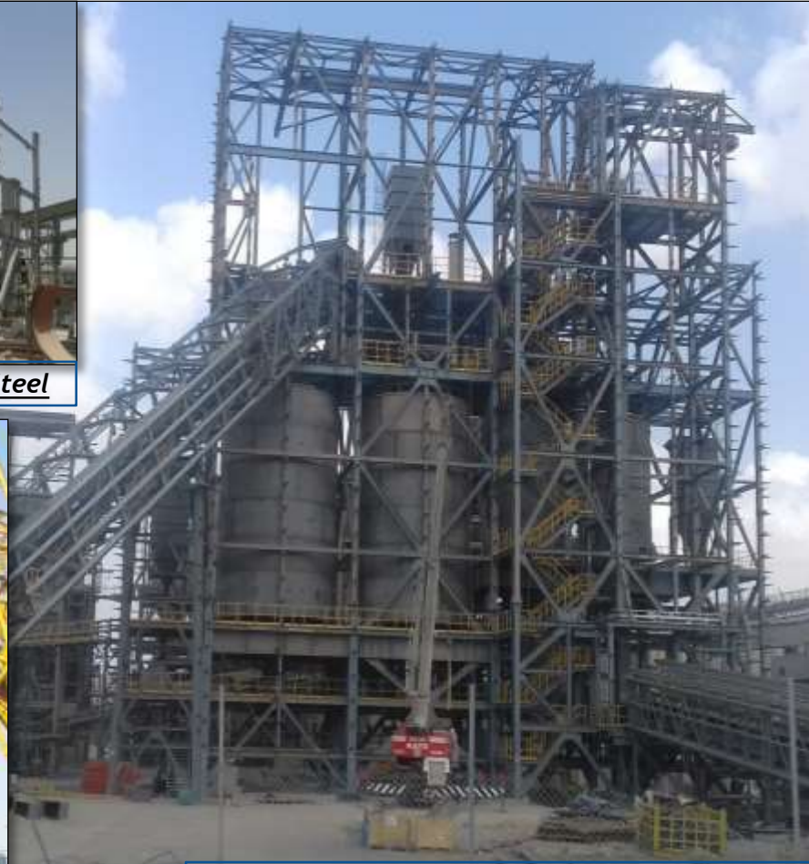
Erection of 511-Mill Feed Building
