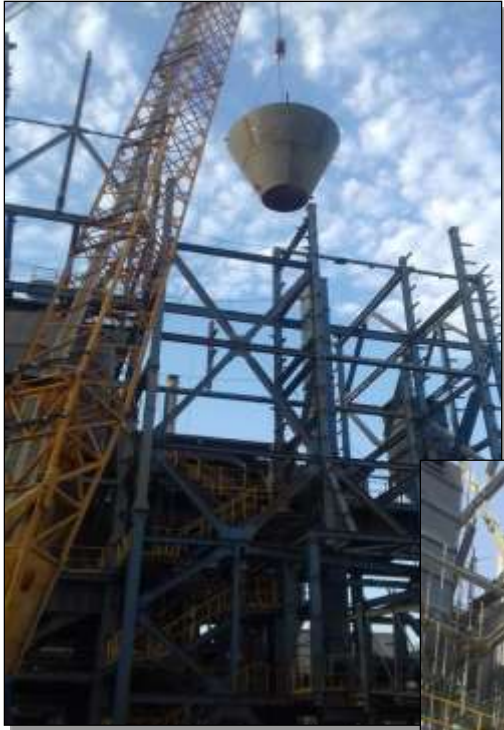
Fabrication & Erection of Bottom Cone of Bins
