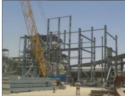
Erection of 511- Structural Steel
