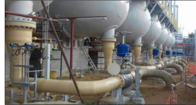
GRP Piping Fabrication & Erection Works in DMPF Area
