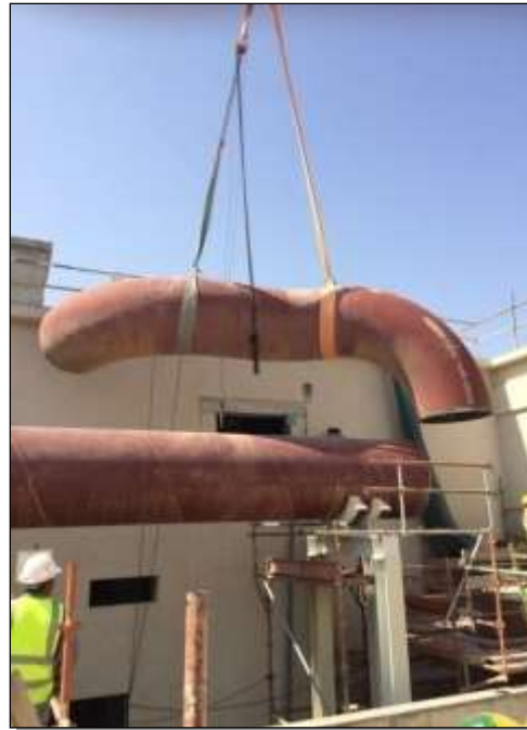
Erection of Prefabricated Pipe Spool at Energy Center
