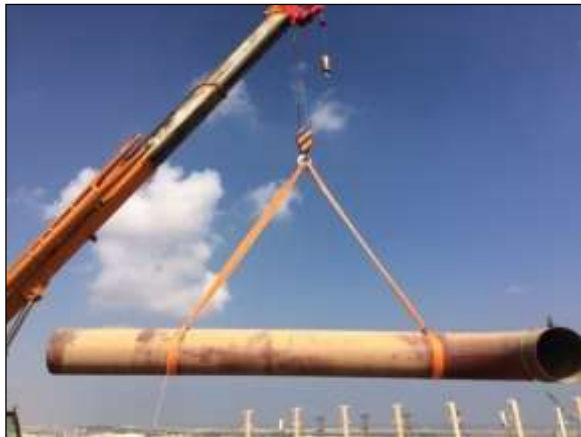
Erection of Prefabricated Pipe Spool at Energy Center
