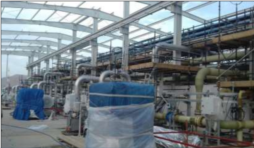
Super Duplex Piping Fabrication & Erection Works in RO Skid Pump Section
