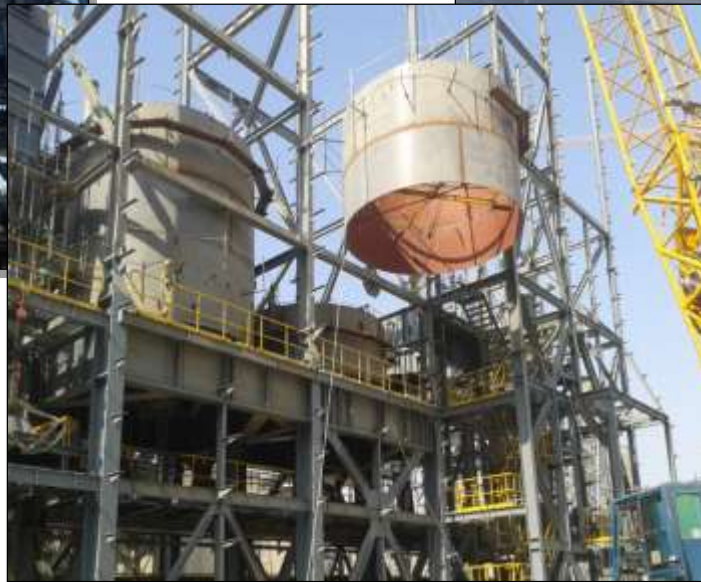
Fabrication & Erection of Bins
